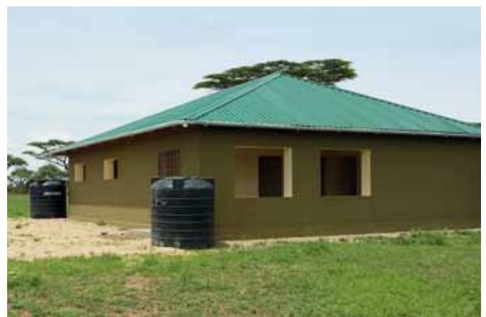
The newly built operations room will act as the nerve centre for monitoring and coordination of anti-poaching operations in the park.
