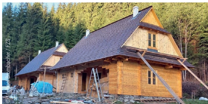
New high quality and ecological ranger houses constructed in accordance with traditional architectural practices were built in Ukraine's Verkhovynskiy National Nature Park, near the Romanian border. A second building functions as a guesthouse for tourists.
