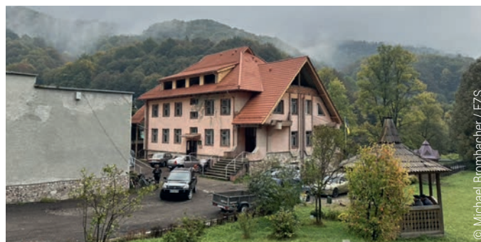
The main administrative building in the Carpathian Biosphere Reserve is currently being renovated. It had a leaking roof which was repaired and replaced.
